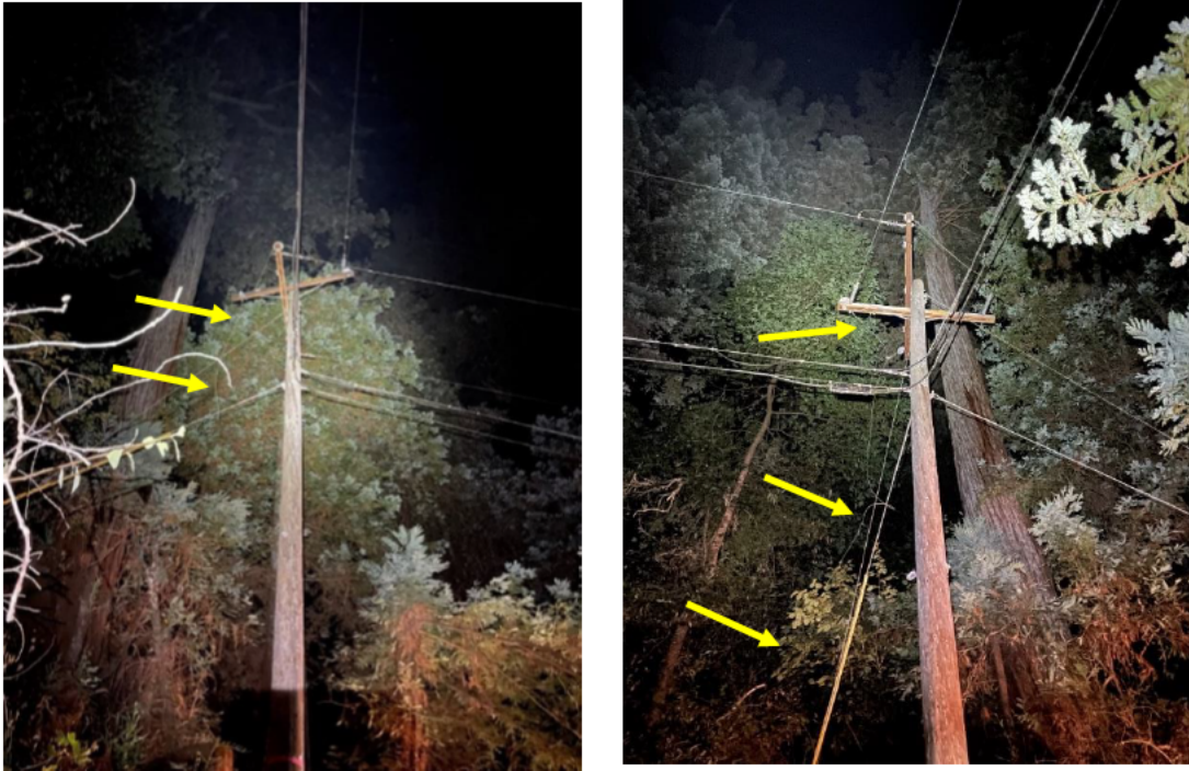
Figure 5 Photographs of top of Pole #1 showing broken conductor (indicated with arrows). Source: Troubleshooter, taken on October 4, 2024.
